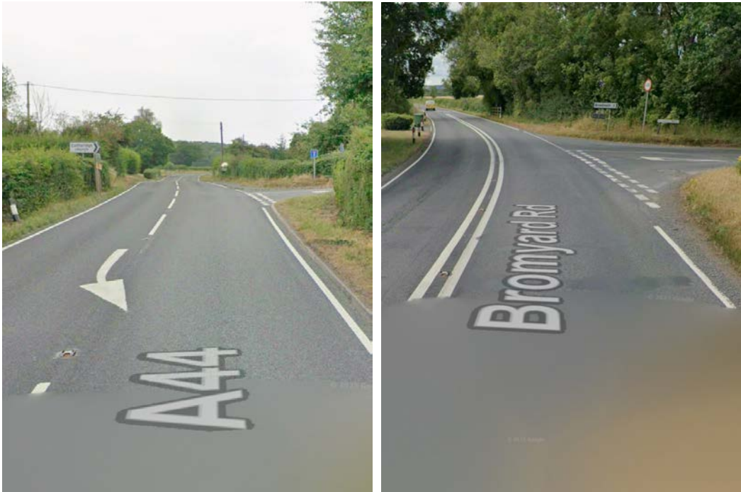
Figure 22 - Accesses to the A44 in Cotheridge
