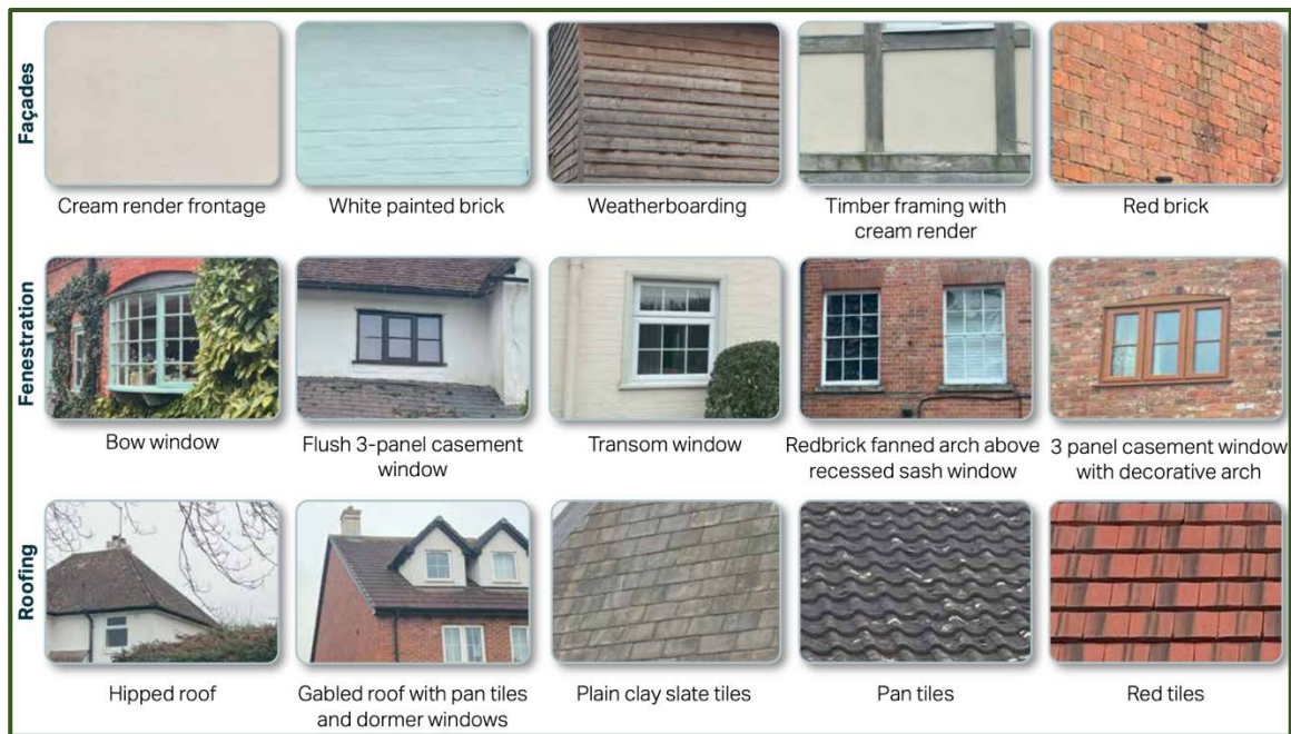
Figure 9 – Local Roofing, Window and Façade Details
